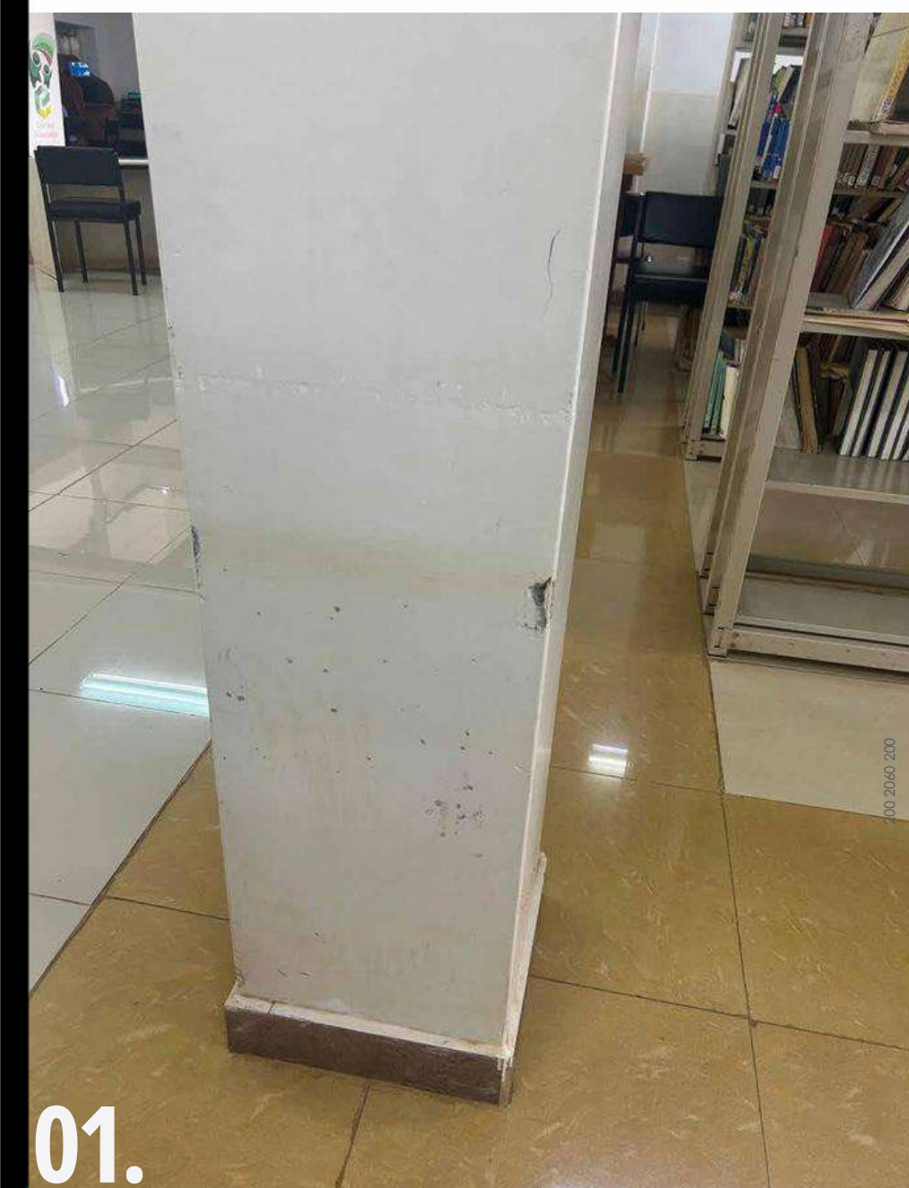
SURFACE IMPACT CRACK
