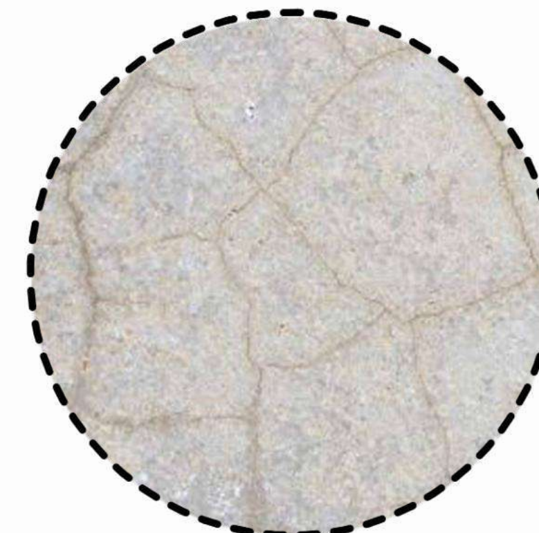
SHRINKAGE CRACKS
