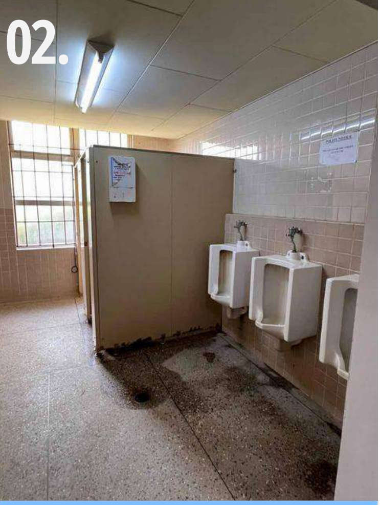
SIGNIFICANT MOISTURE DAMAGE IS VISIBLE AT THE BASE OF THE PARTITION WALL. THE FLOOR SHOWS EXTENSIVE WET PATCHES AND STAINING AROUND THE FLOOR TRAP, SUGGESTING RECURRING DRAINAGE OVERFLOW OR LEAKS.
