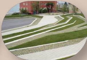
Precast drainage slab
