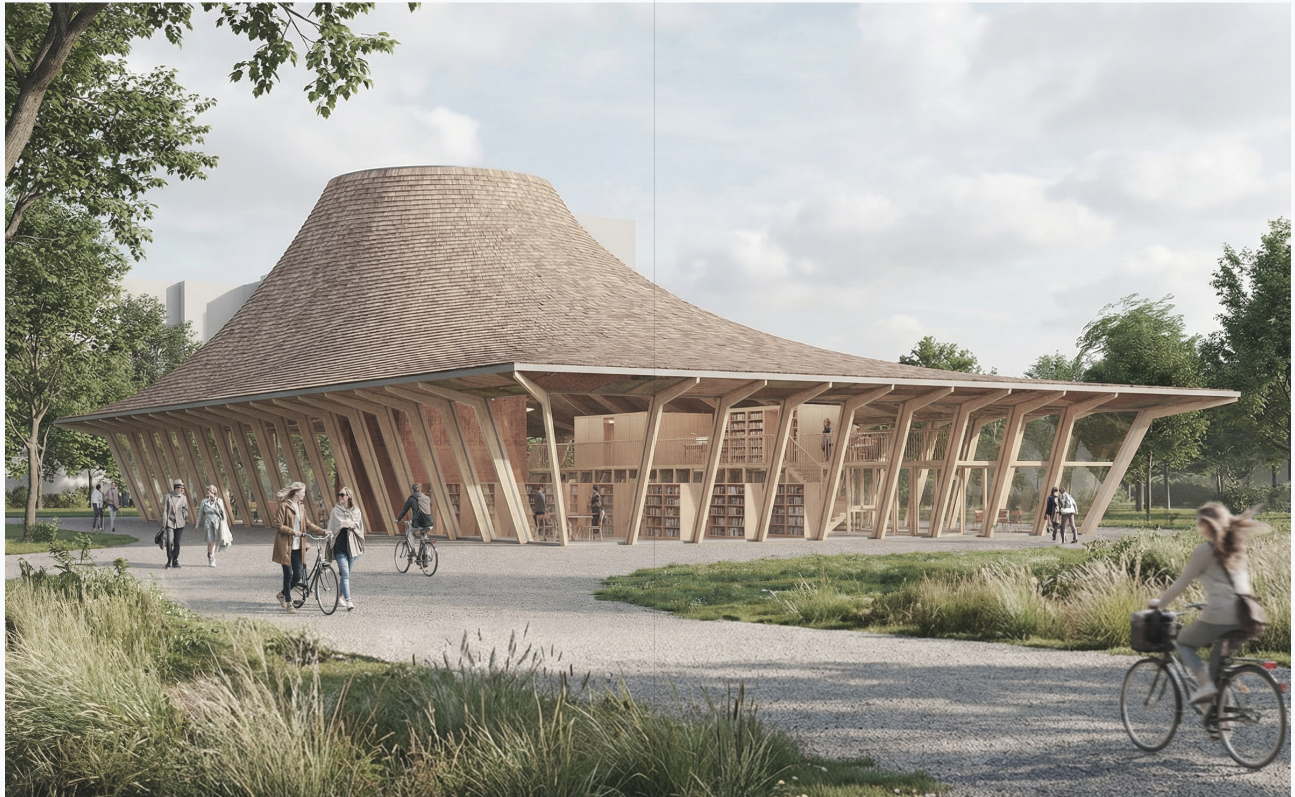
Viewed from the southeast. The angled façades accentuate the sense of tension embedded within the roof form, while their openness creates a strong relationship between the building and the surrounding park landscape.
