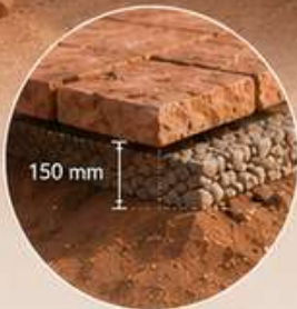
EDGE DETAIL The walkway is lightly elevated above the desert while remaining reversible and non-invasive.
