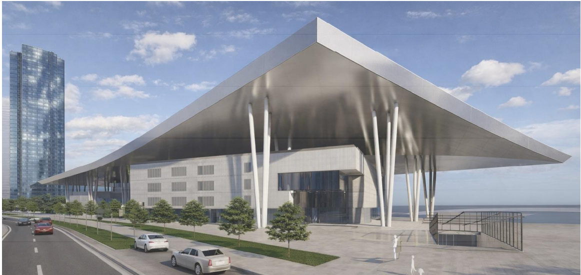
Fig. 1.13. Visualization. Main facade. View from the central plaza
