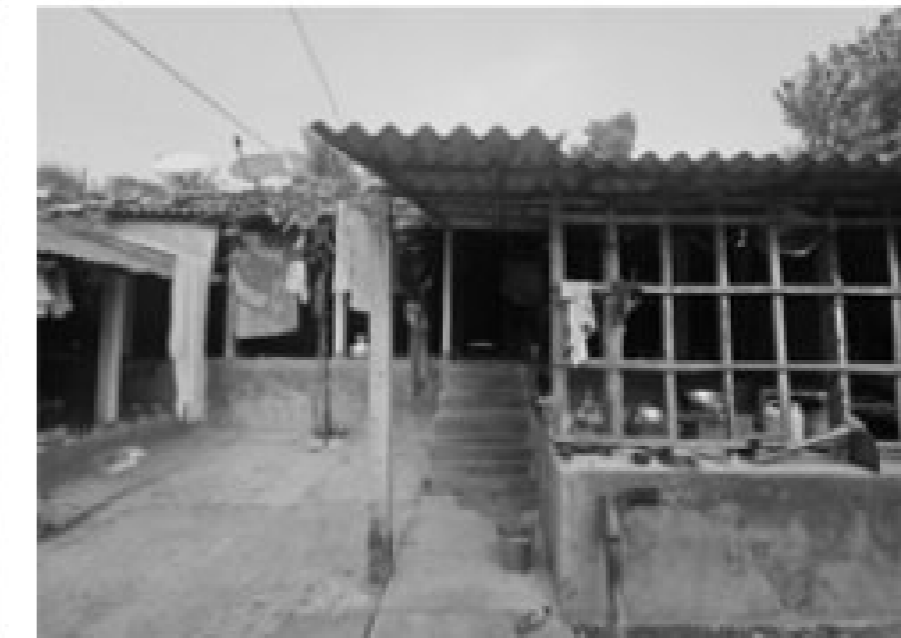
Img. 32: Most kutcha houses are rebuilt using pre-fabricated concrete columns, and daily used spaces are constructed firmly
