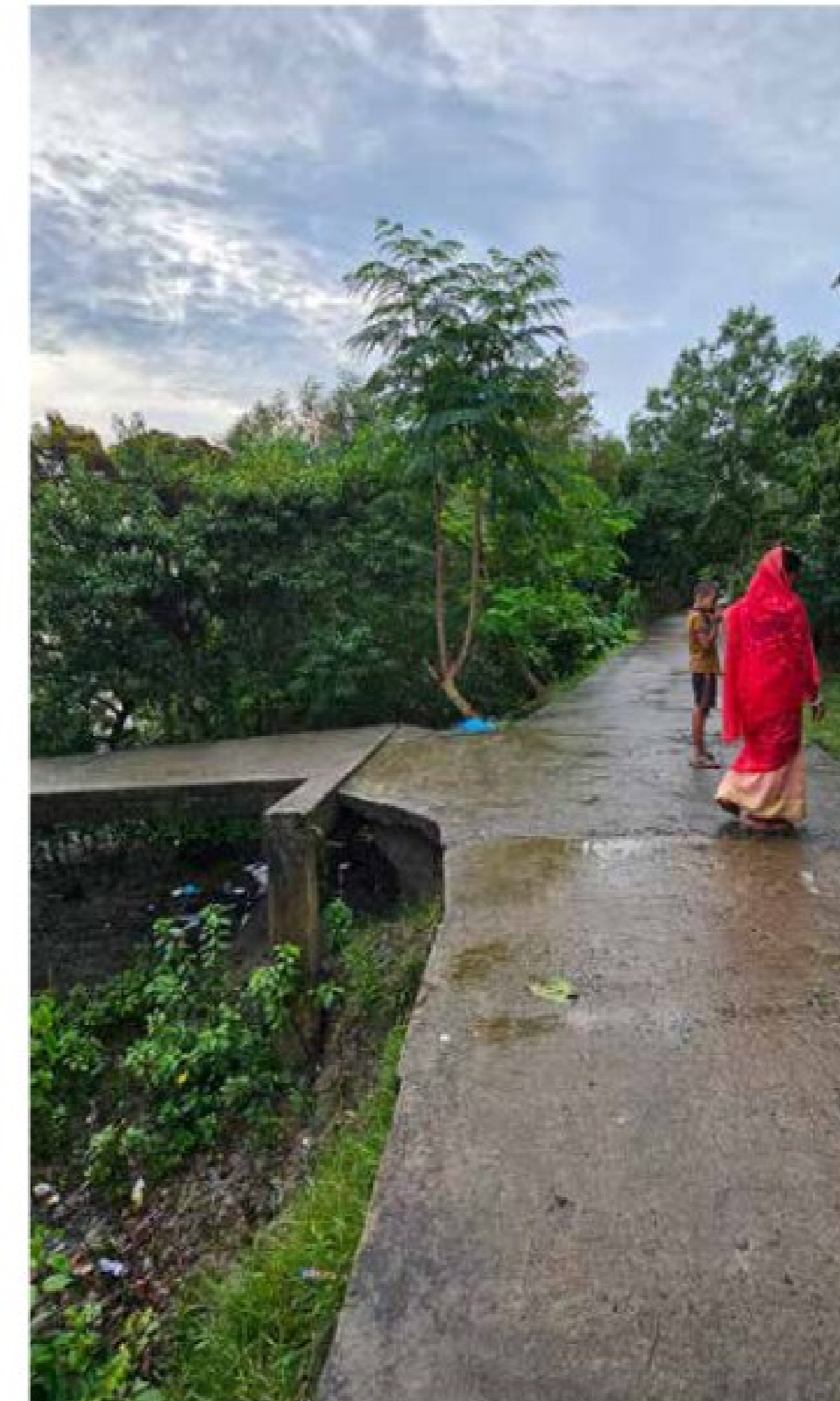
Img. 16: Raised embankment path functioning as access route and flood edge.
