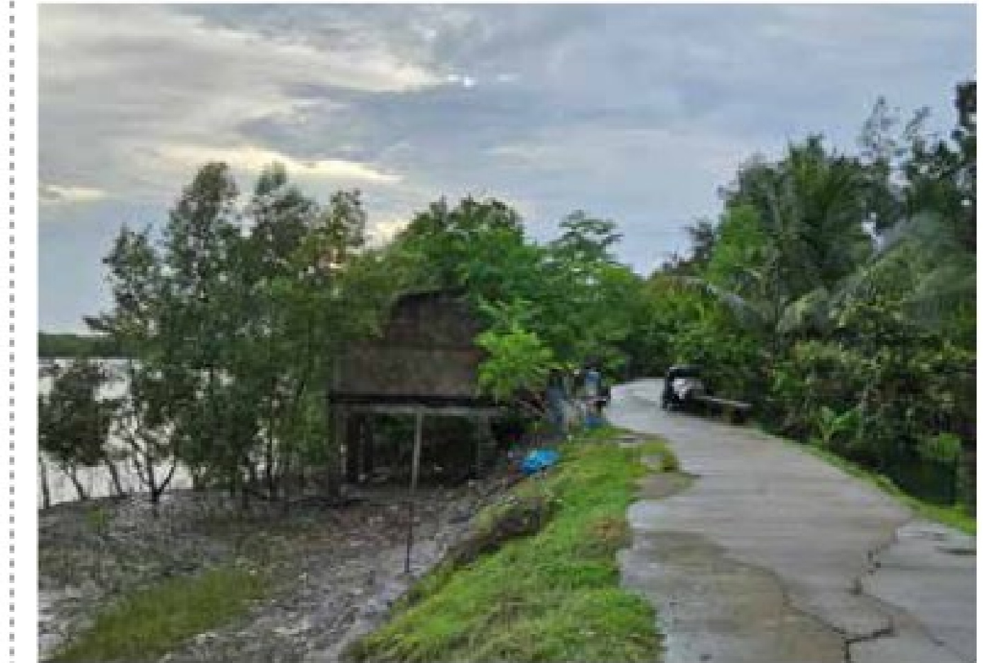
Img. 05: Shops raised on stilts near the river edge, allowing everyday activities to continue despite changing water levels.
