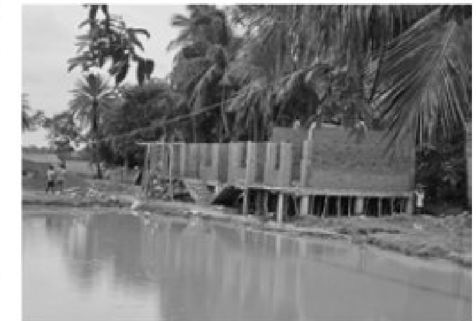
Img. 36: Newly built semi-pucca houses are constructed on raised plinths
