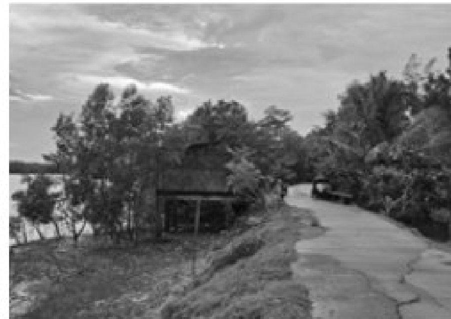
Img. 26: Embankments are considered as the highest point, which protects the island from flooding
