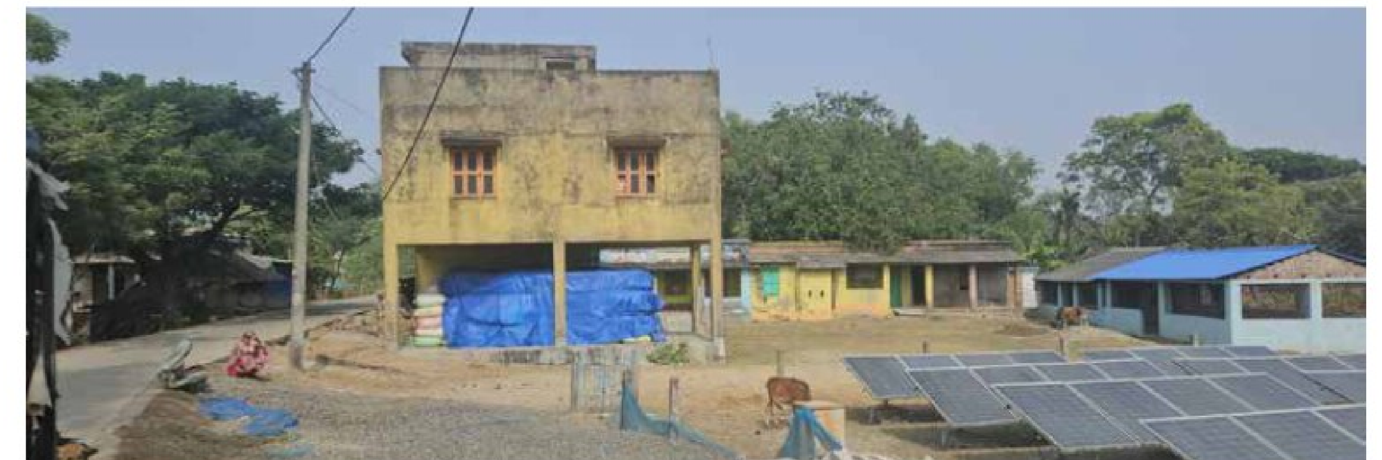
Img. 23: Anpur Flood Shelter, currently used as place to store construction materials
