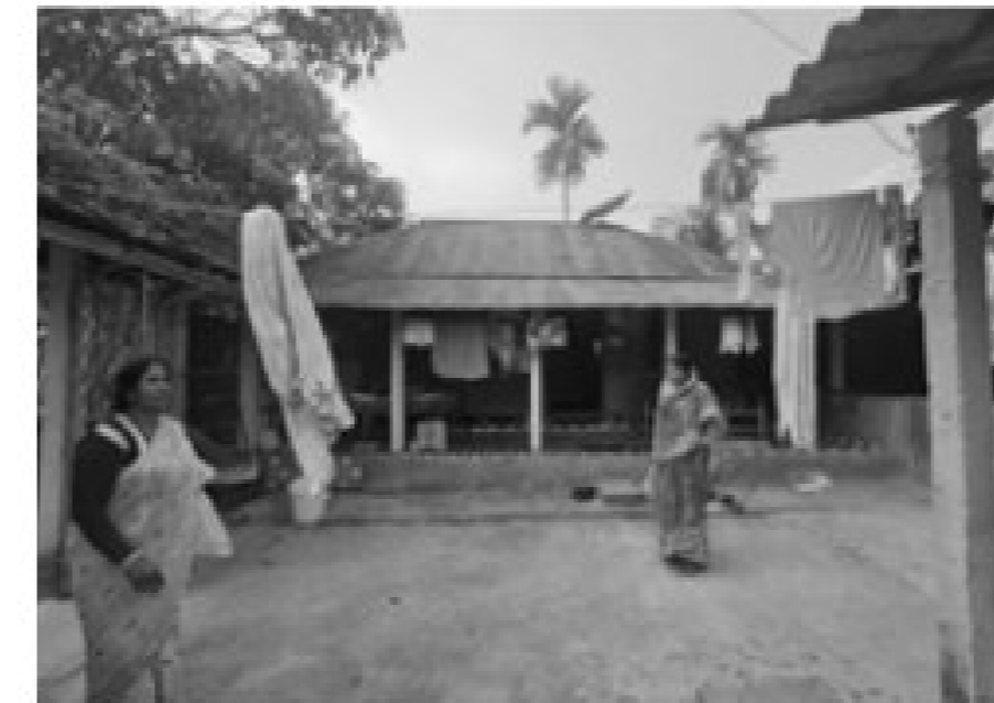
Img. 31: Most kutcha houses are either made using mud, pre-fabricated columns or bamboo, with thatch or corrugated sheets for roofing
