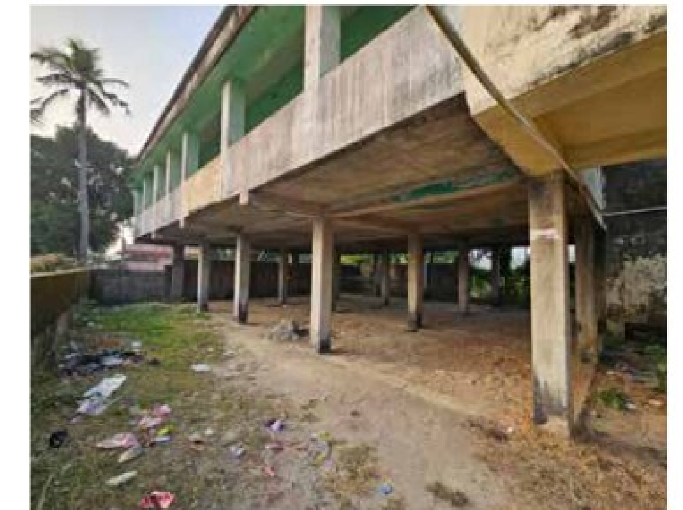
Img. 22: Rajat Jubilee Flood Shelter in Anpur (ground floor)
