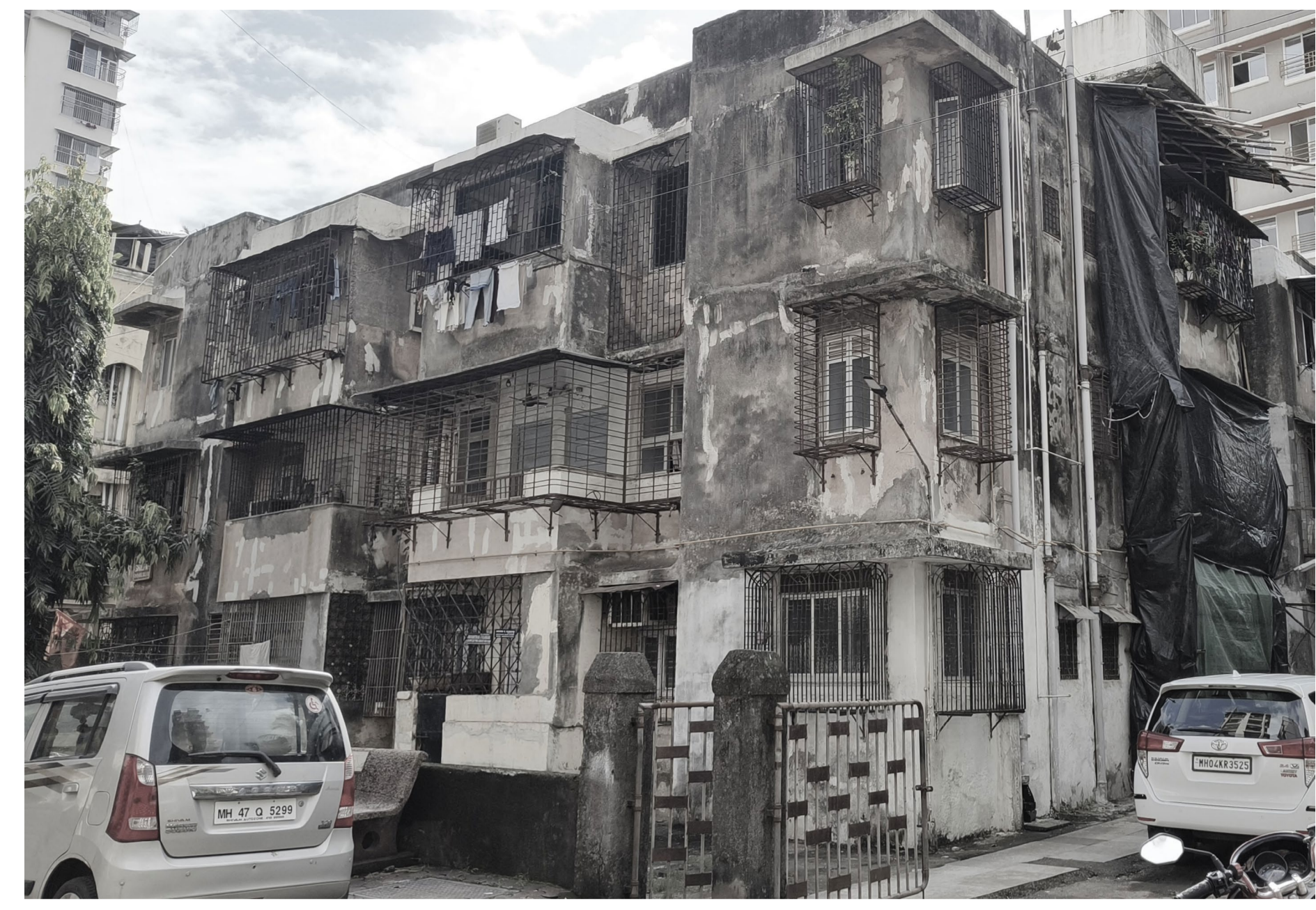
Existing on-site building proposed for redevelopment.
