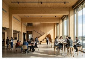
Internal of runner main pre-function area (from 11m GLT beams), creates column-free, flexible space — integrated stairs with AirStairs (source 4.1).
