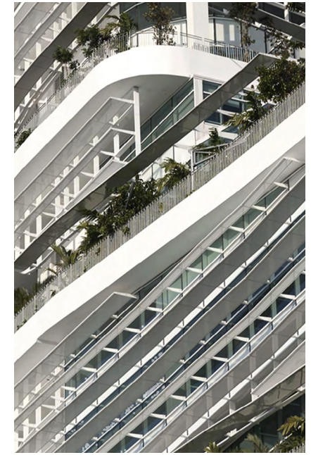
Figure 49. Facade detail of the Solaris building. Source: Charles Moxham, 2011.
