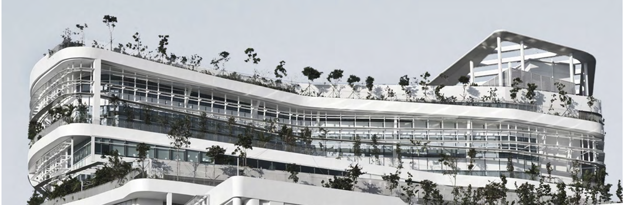
Figure 47. View highlighting the roof of the Solaris building. Source: Charles Moxham, 2011.
