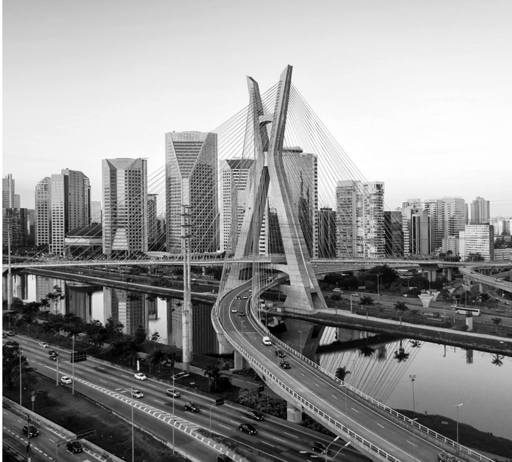
Figure 9. São Paulo Cable-Stayed Bridge. Source: Ecrie70, 2023.
