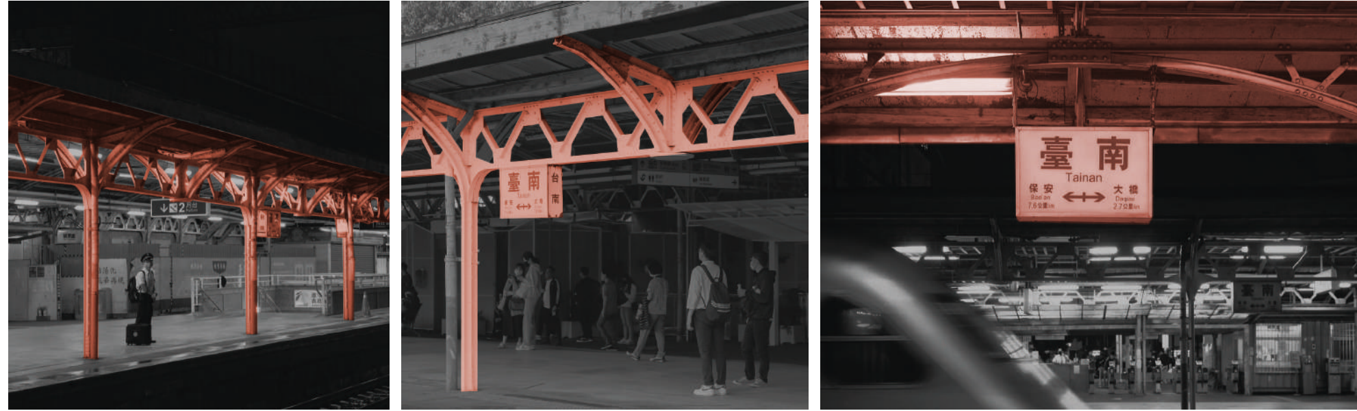
Tainan Station Current Platform Shed
