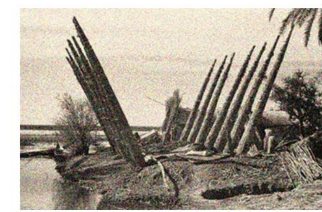
They bind the independent arches into a unified grid. This structural tie prevents lateral buckling of the main arches and ensures lateral wind loads are distributed evenly across the entire framework
