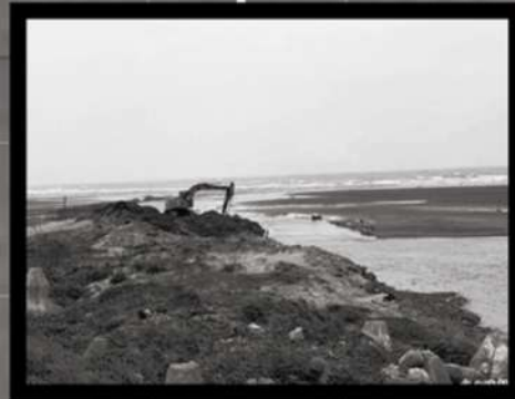
Coastal Engineering and Shoreline Modification
