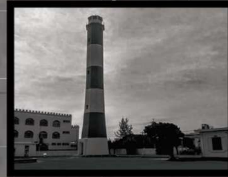
Gaomei Lighthouse Completed
