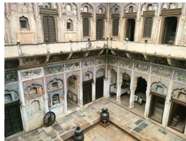
Inner Courtyard of Haveli
