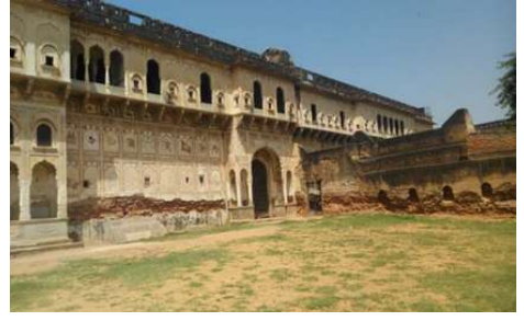
FRONT VIEW OF THE HAVELI
