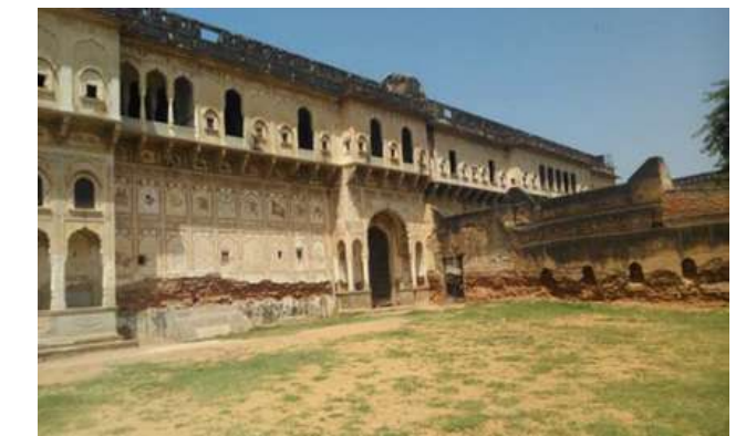
FRONT VIEW OF THE HAVELI
