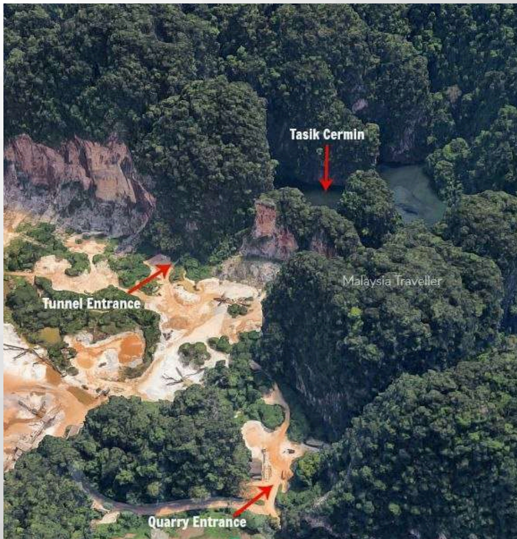
Figure 4.3: An overview of the site
