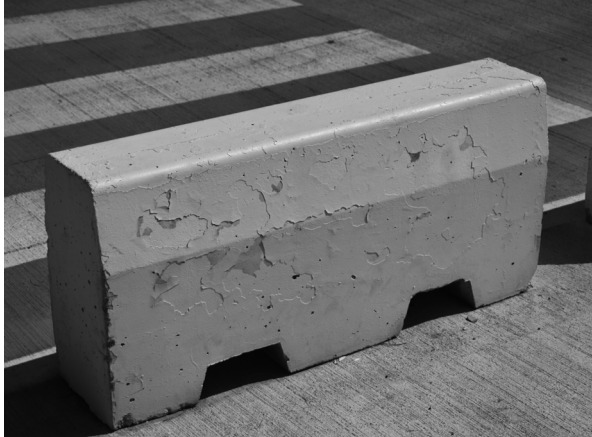
Separation concrete barriers
