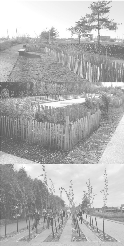
1.2.3. Cuts into asphalt allow the start of a framework and space for planting with only moderate intervention, 2017
