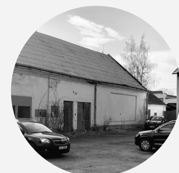
White lime render and clay roof tiles
