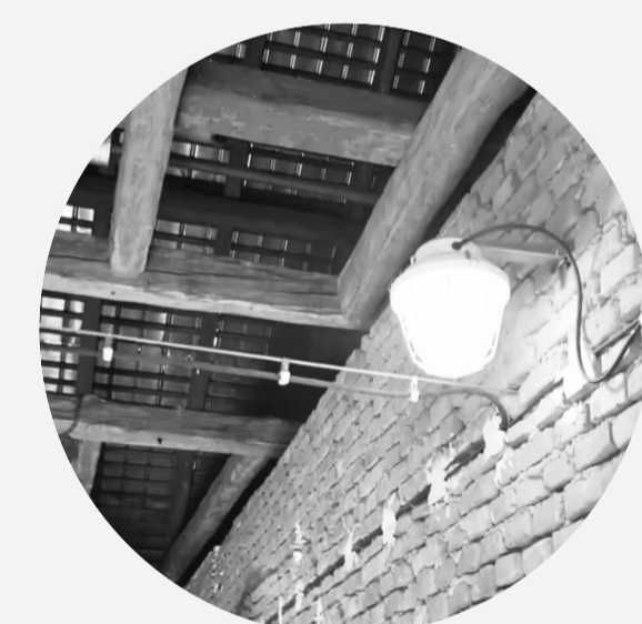
An interior featuring exposed timber roof trusses and brick walls
