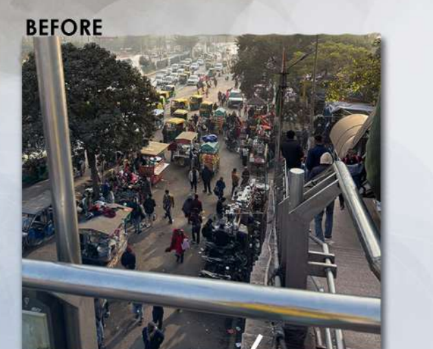
DEDICATED PLATFORMS ORGANIZE SCATTERED STALLS TO CLEAR ROAD AND BRIDGE CONGESTION, CREATING A FLEXIBLE SPACE THAT TRANSITIONS FROM A MARKET FOR COMMUTERS BY DAY TO A KIDS RECREATION ZONE AT NIGHT
