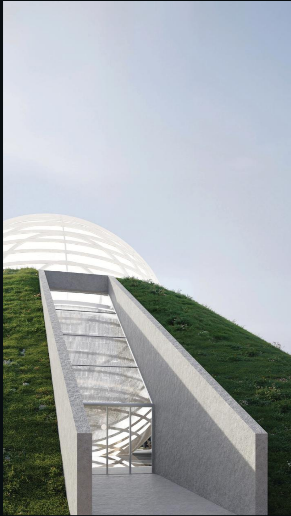
DETAIL OF THE BUILDING ENTRANCE
