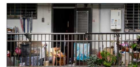
Iron fence / Iron railings
