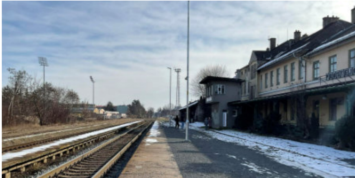
Local railway station at present (northern part)
