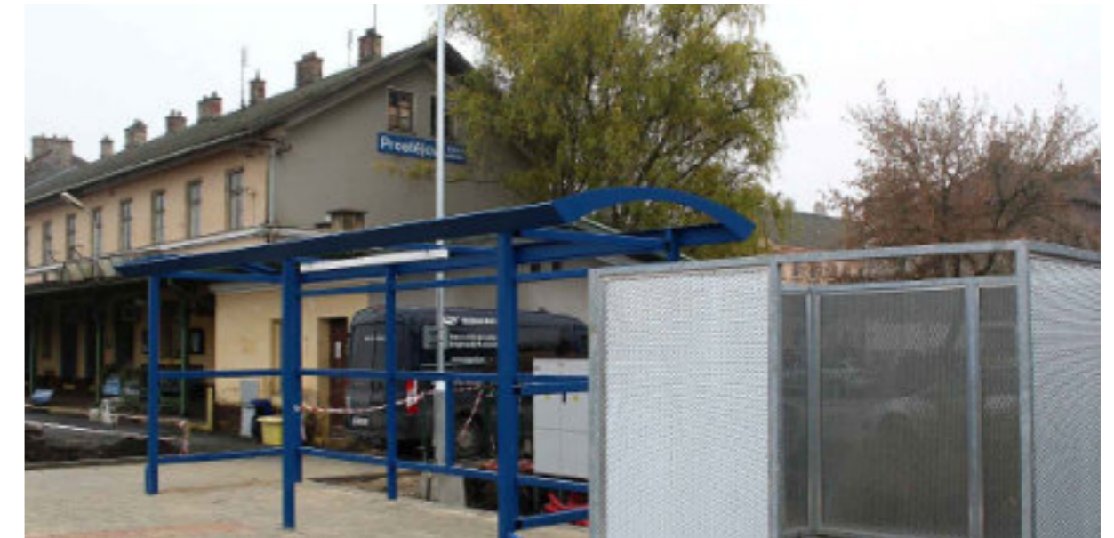
Local railway station, installation of the new train stop 2025
