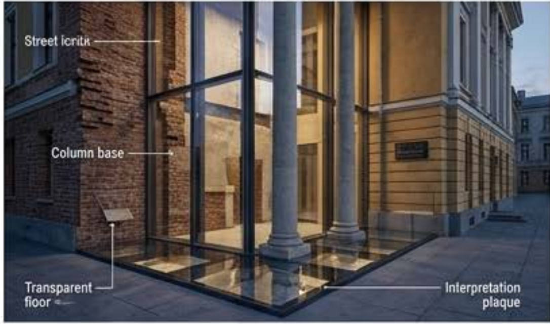
VISIBLE CONFLICT SCARS PRESUMED & INTEGRATED... old brick, new steel and glass, preserved stone columns, and interpretation plaque
