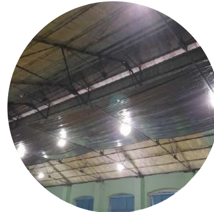
TWO-WATER COVERING OF CORRUGATED SHEET, SUPPORTED BY METALLIC BRACKETS.
