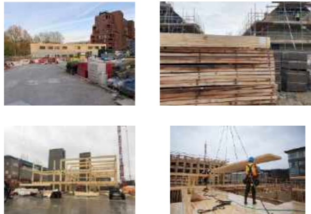
Stages of wooden house constructed
