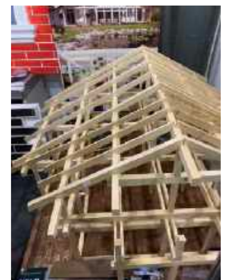
Structural elements - photos made by author.
