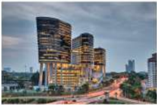
SPRM OFFICE BUILDING SPRM OFFICE IS LOCATED AT PUTRAJAYA. THIS OFFICE BUILDING IS A UNIQUE BUILDING AS IT USED OUTRIGGER STRUCTURE SYSTEM.
