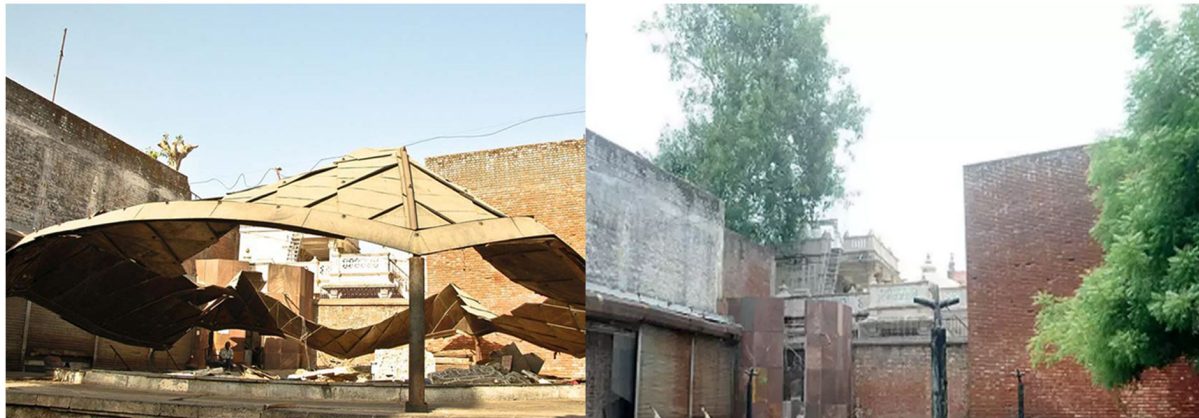
The below picture on the left shows the leftover dome till 2017 and on the right shows the recent ones with just metal piers left intact.
