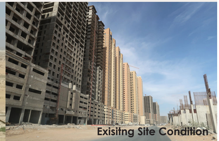
Existing Site Condition
