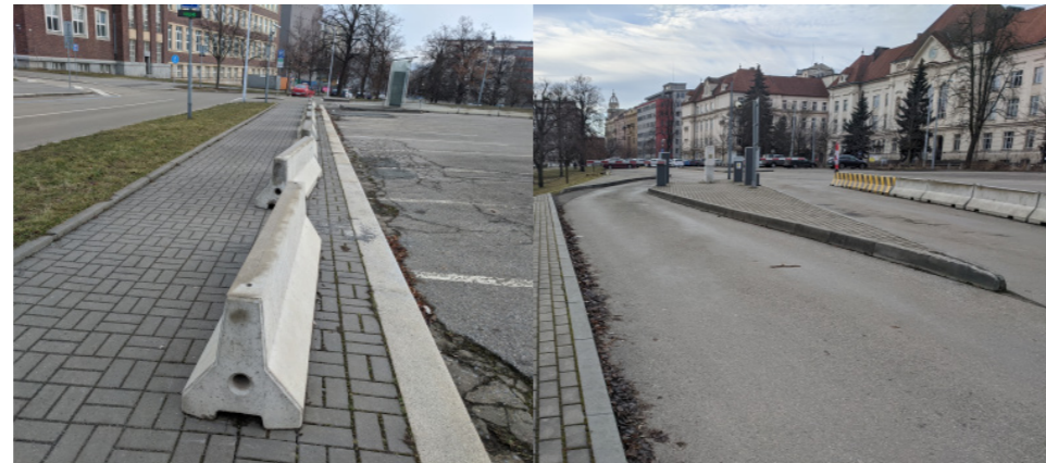
view, too much concrete in the area makes this place uncomfortable hot in summer days (photos - February 2021)
