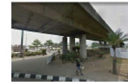
view of eko bridge
