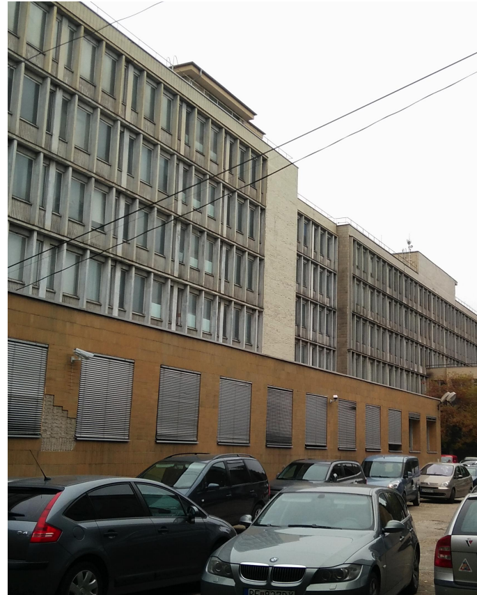
facade of Faculty of mechanical engineering
