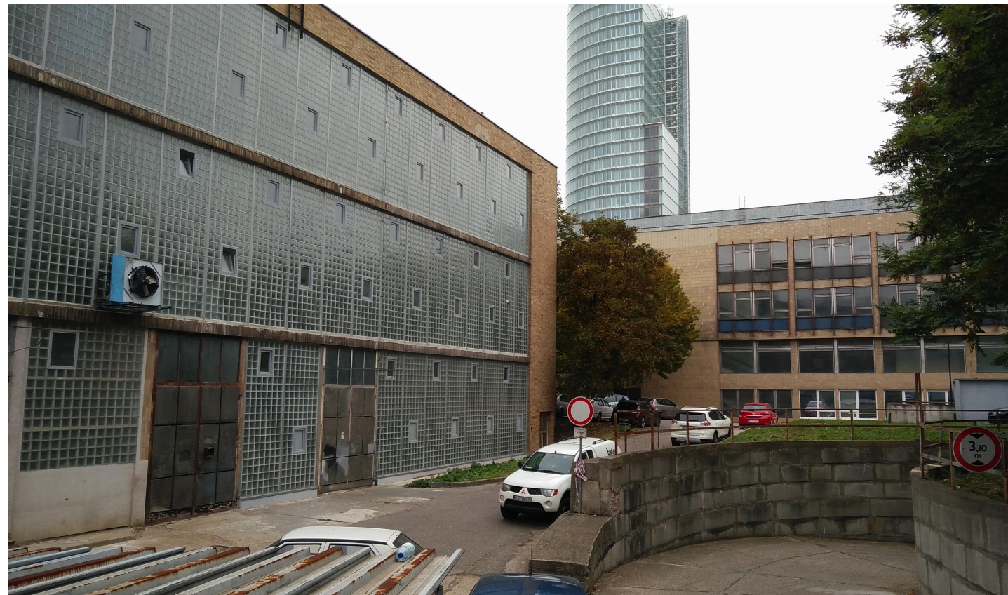
Facade of Object of heavy laboratories and Faculty of civil engineering
