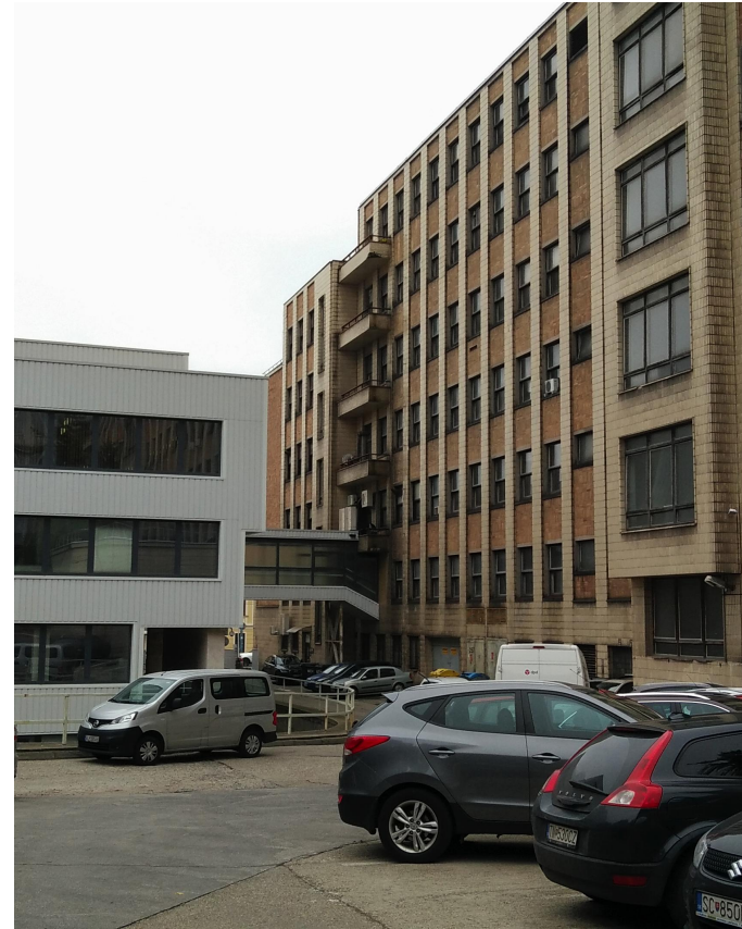
facade of Faculty of chemical and food technology
