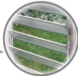
Louvered window (Toilet)
