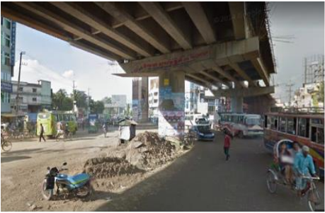
Fig : Bahaddar Hut Junction
