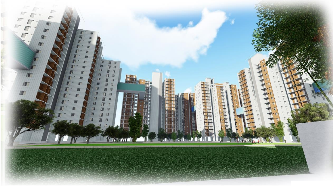
VIEW FROM ENTRY
