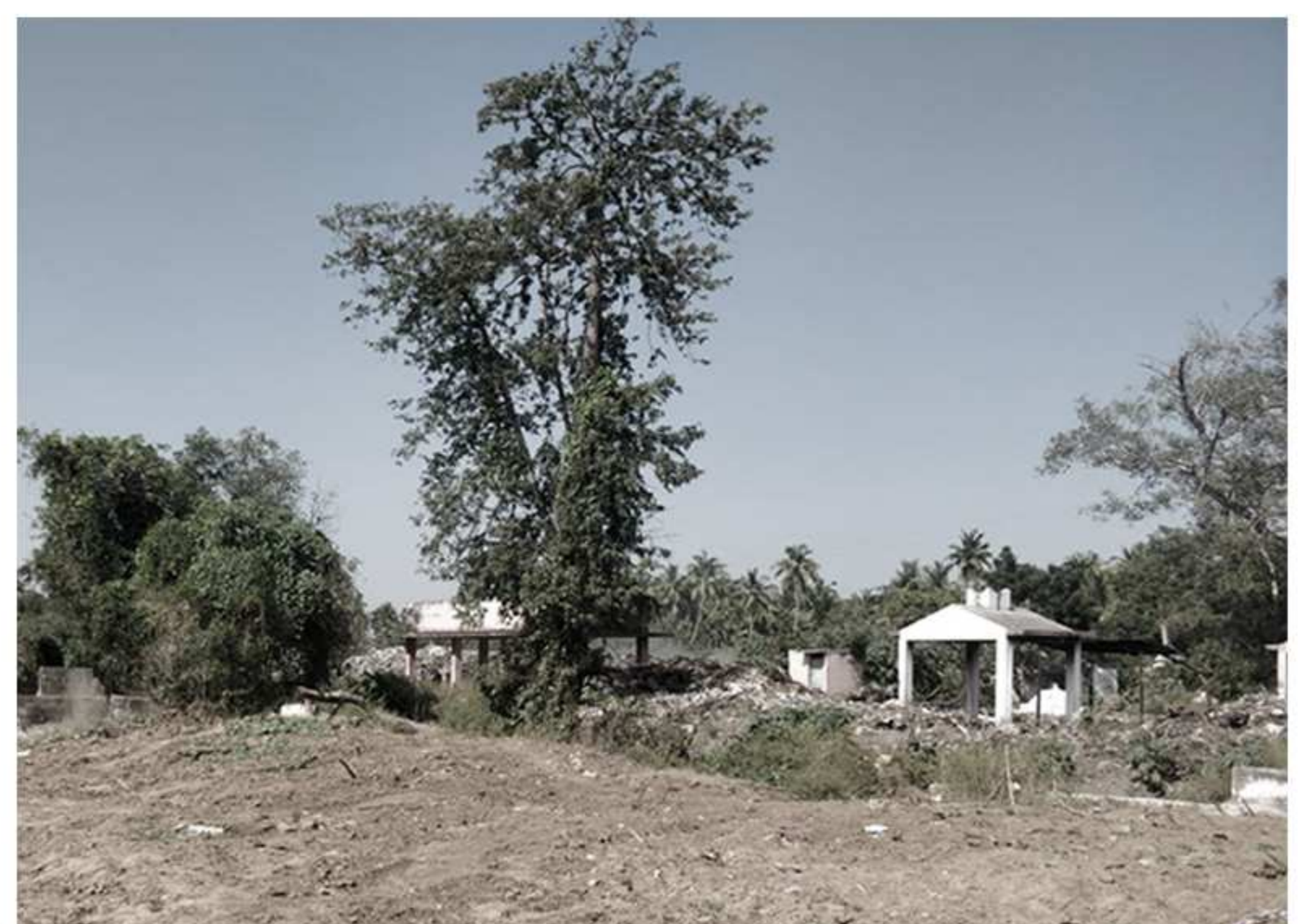
Existing crematorium structure
