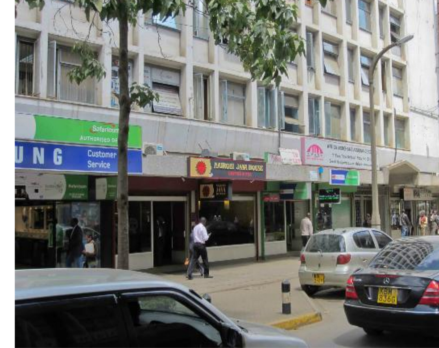
Shops with large display windows
